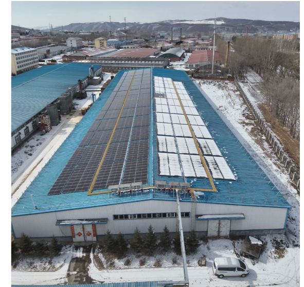
182 單晶單玻 545W 光伏元件 182 Single-crystal Lattice Single-layer 545W PV Component
